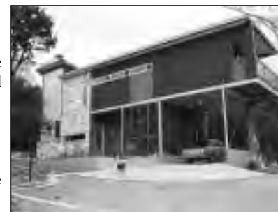
The air conditioning in this modern Westlake home starts in the ground with a geothermal system and ends in a Koi pond, fed by the condensate line.
