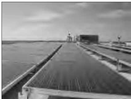
The McKinney Green Building in McKinney, TX is a 42 kW system
