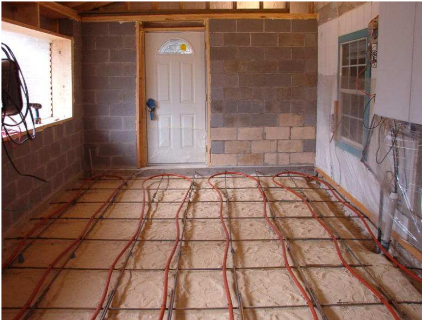
Solar in-floor radiant heat under construction.
