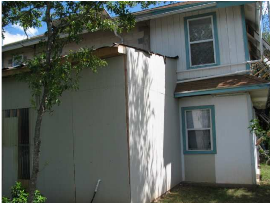
5,000 gallons of rainwater are housed in this enclosure.
