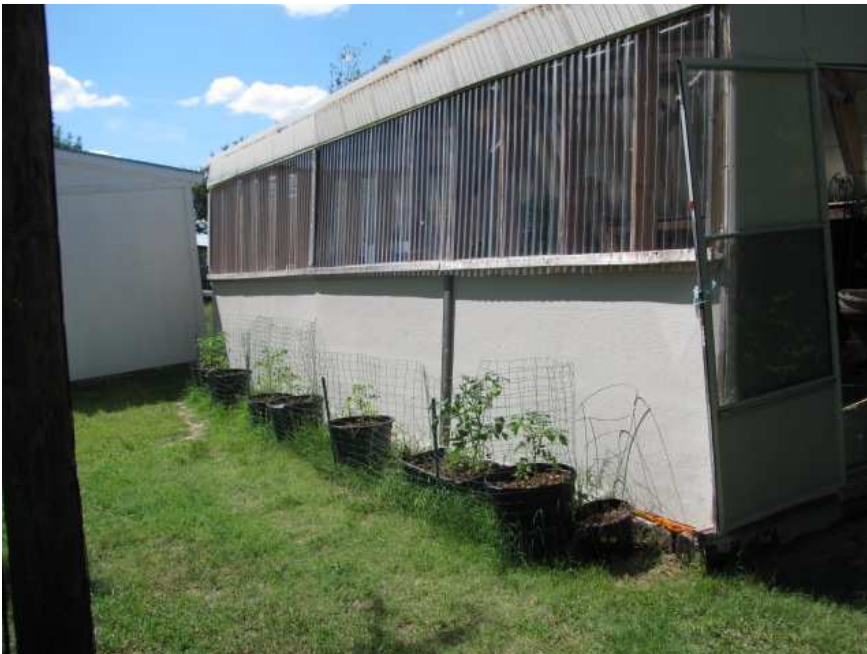
Translucent panels allow sunlight to enter the greenhouse.
