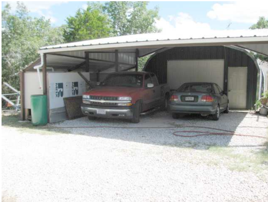
Carport rainwater capture. Enclosed area (behind green barrel) is storage.
