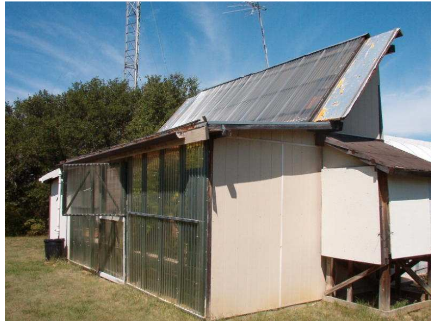
The solar greenhouse. Windows allow cool air in during summer.
