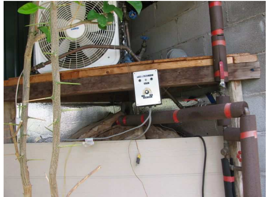
Home-made electronic temperature controller. Note the pipe insulation!
