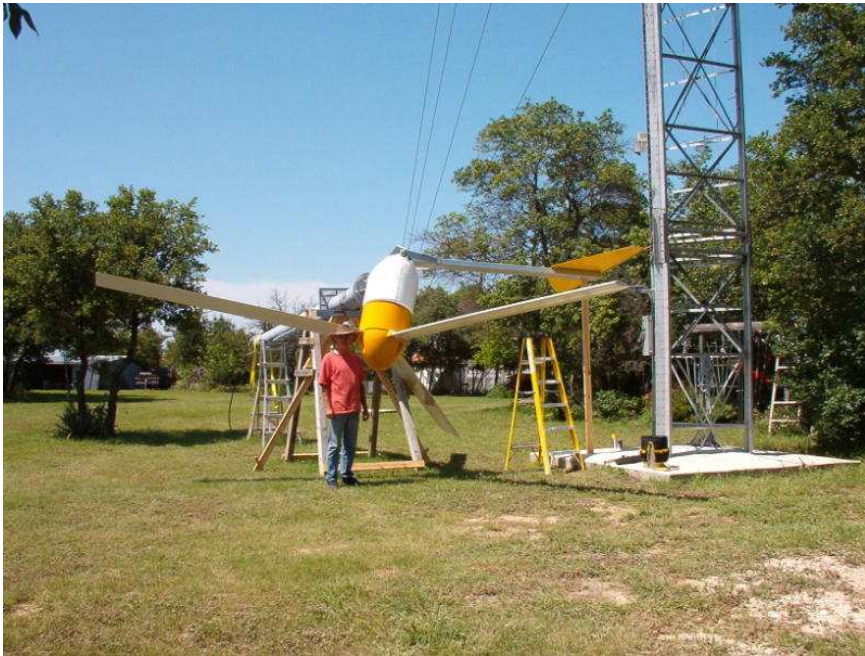
The 10,000 watt Bergey wind generator. Note its size compared to Mike.
