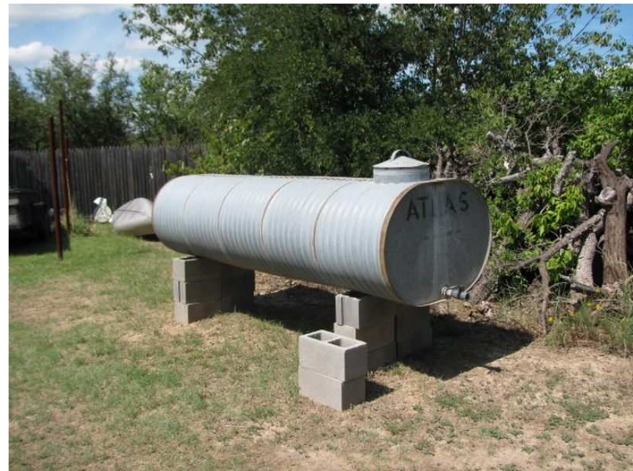
500 gallons of water storage capacity ready to be installed..
