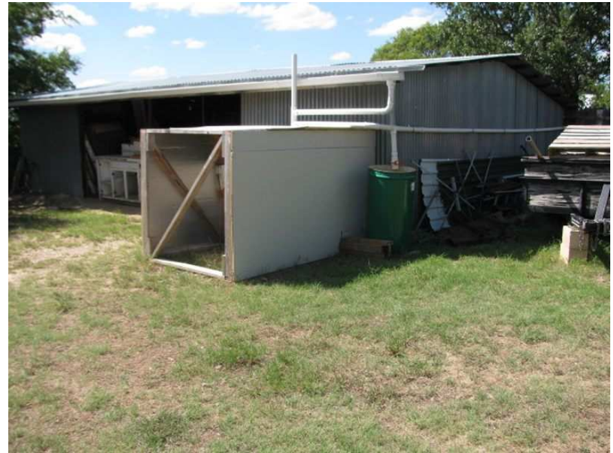
Rainwater capture on the shed.
