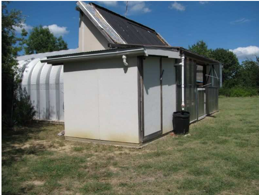
Rainwater capture on the greenhouse. (Black barrel.)
