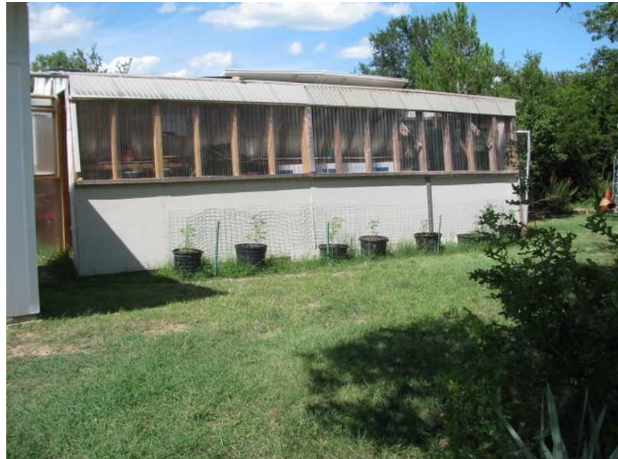
A vent on the greenhouse roof opens to allow hot air out in the summer.
